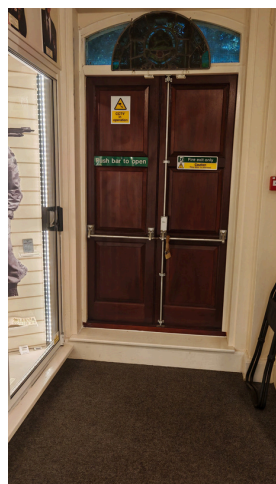
The fire escape
